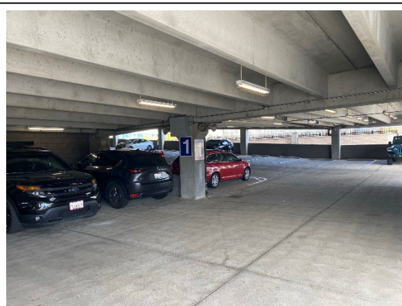
The existing parking structure features a one-way circulation system. Therefore, it would not be possible to continue operation of the parking structure during construction activities.
